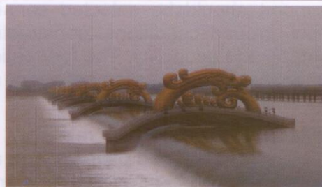
Plate 2: Taoyuan Rubber Dam Project
