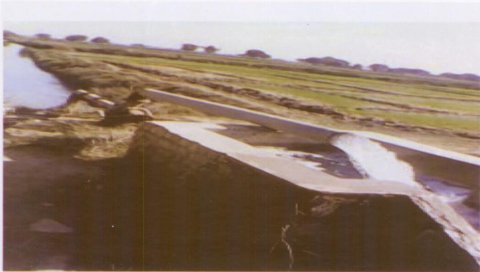
Plate 6. Another View of Pumping Drainage Water for Irrigation to the Crop Experiments
